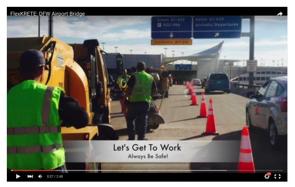
**The Dallas-Fort Worth International Airport** north entry to the Terminal A bridge had 80+ potholes that spanned the nearly 300 feet long crossover. It's a great example of how other repair materials failed but is the ideal setting to illustrate the advantages of the FlexKRETE's fast-set, high-strength, and long-lasting Concrete Repair System.
